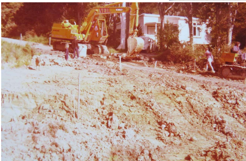
The Roadworks at the intersection of Brownie Rd
