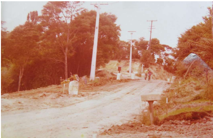
Road works towards Laingholm Beach and Store Janet Place
