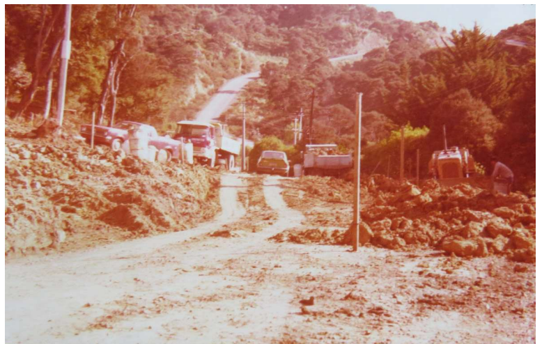
Roadworks from Brownie Rd towards Fawcett Rd up towards Helios PI
